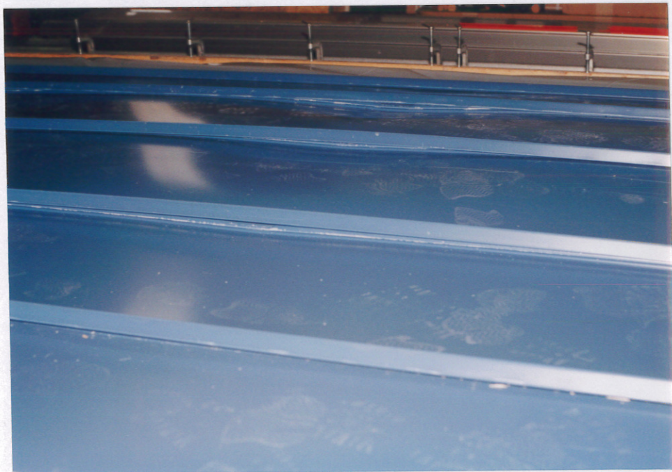
PHOTOGRAPH J SEPARATION OF PANELS
